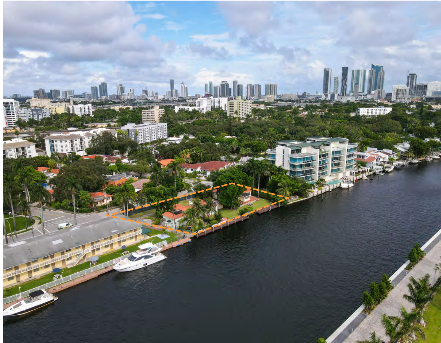
Aerial photo of site looking east
